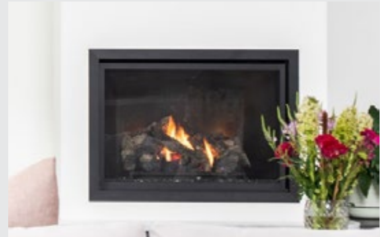
Example of firebox with 50mm trim & non combustibile wall sheeting
