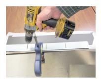
5. When installing the face brackets, secure the brackets through the holes drilled using the template.
