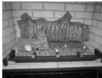
Figure 8: Left Log Installed
