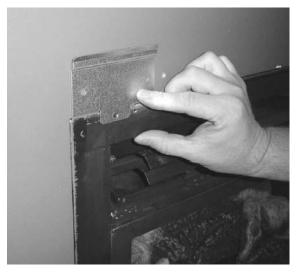
2 Use the included 9/64" drill bit to drill a hole through the front of the fireplace directly behind the lower hole on the bracket (see photo below). Make sure to penetrate only one layer of steel. Use one of the included screws to secure the bracket to the fireplace (see photo below).
