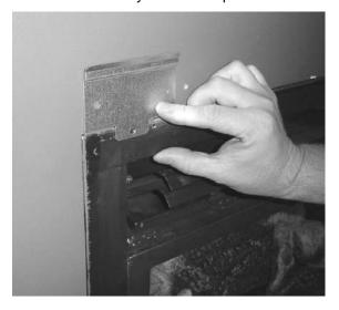
Use the included 9/64" drill bit to drill a hole through the front of the fireplace directly behind the lower hole on the bracket (see photo below). Make sure to penetrate only one layer of steel. Use one of the included screws to secure the bracket to the fireplace (see photo below).
