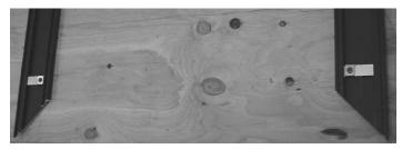
Once all of the spacers and "L" brackets are fully inserted, carefully align the trim, making sure each corner butts correctly to the adjoining piece. Tighten the set screws to secure the trim pieces together (see photo below).
