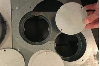
10. Remove the left, top layer, cover plate. Turn it over and then reinstall it in place of the right cover plate removed in step 7. Replace all screws so there are no holes left in the top of the fireplace.
