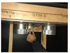
Remove the right cover plate (with the single knockout) from the top of the fireplace and discard it.
