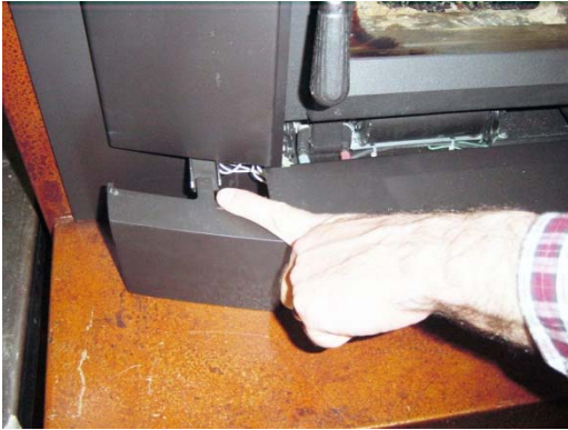
Figure 17: Attaching the lower face
