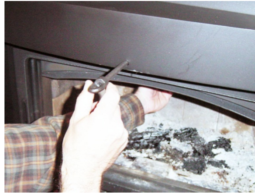
Figure 24: Attaching the extension rod
