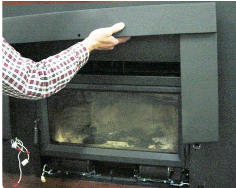
Figure 9: Attaching the face
