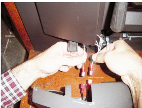
Figure 15: Connecting the bottom left wires
