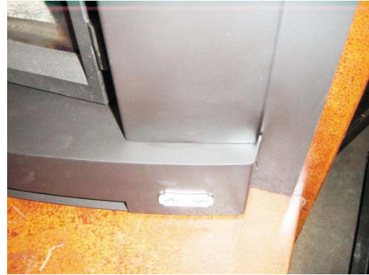
Figure 18: Face aligned flush with the insert
