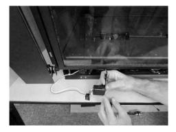
Insert the switch into the bracket, and then attach the bracket to the insert. Secure the wires to the insert, making sure they do not contact any hot or moving components (use lock-ties if necessary).
