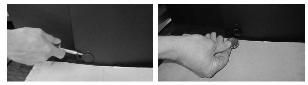
6 Route the Molex plug on the wiring harness through the hole on the right side of the insert. Then reach in from the front of the insert and pull the Molex plug forward.
