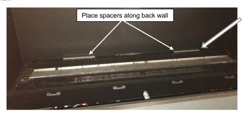
4 Install the rear fireback(s). Insert one end of the fireback through the firebox opening. Move it all the way to the side of the firebox and carefuly move it deeper into the firebox until the opposite end of the fireback clears the opening. Once the entire fireback is in the firebox, manuever the fireback parallel to the back of the firebox.
