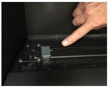
2 Spread an even layer of crushed glass over the media tray and burner. The glass must be only 1 layer thick on the burner but can be 2 layers thick on the media tray. **Make sure no glass is in the pilot area** indicated in the picture below.
