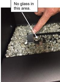
3 Make sure the rear and end air channels are free of crushed glass. Use a screwdriver to clear this area.
