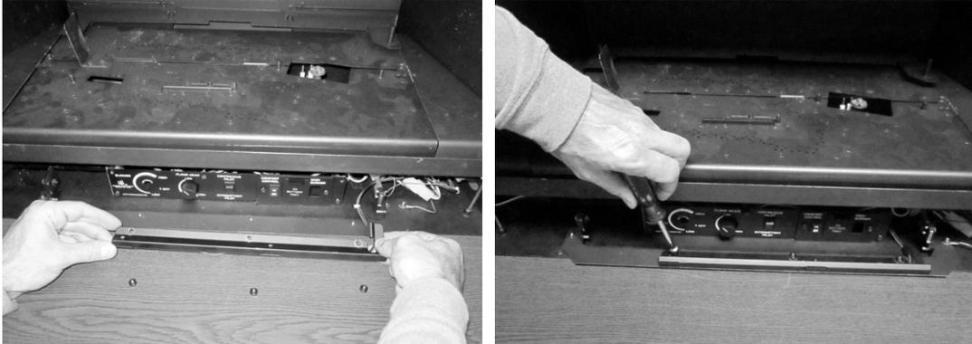
The switch bracket attaches to the Shadowbox face. Remove the two lower inside nuts (see photos below). Place the switch bracket over the studs and secure using the nuts removed earlier.
