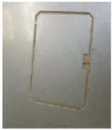
(b) Pry the knock-out forward (use a screwdriver or pliers).
