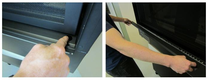
2. Remove the three screws holding the screen in place (1/4" nutdriver- magnetic driver recommended). Then pivot the screen down slightly until the clips on the bottom disengage from the glass frame.
