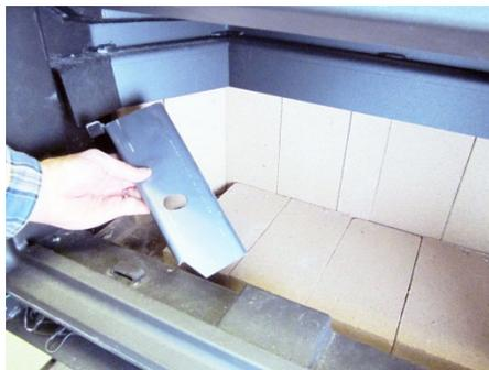
3. Replace the floor firebrick to complete the installation.
