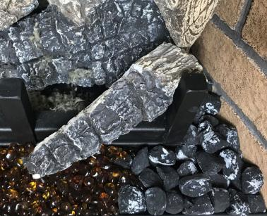
14. The left twig sets on the left most pin on the front left log and the top rests on the left log.
