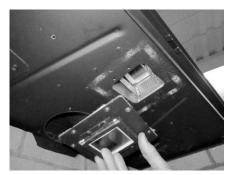
3. Pull down the upper accent light enclosure from the roof of the firebox, as shown below. Note the 3 screws holding the bulb assembly in place.
