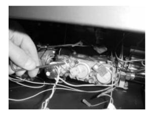
11 Restore the appliance to the correct configuration. Make the gas line connection, bleed the gas line (if applicable), start the heater and thoroughly leak-test all gas connections and the gas control valve.
