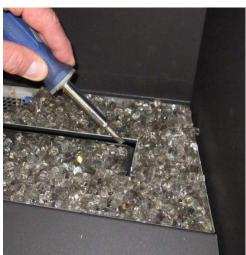
4 Remove the pilot shield to uncover the pilot once you are finished placing the glass.
