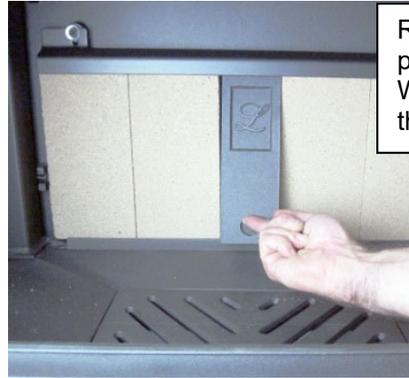
Remove this cover plate (5/32" Hex Wrench) and replace the firebrick.
