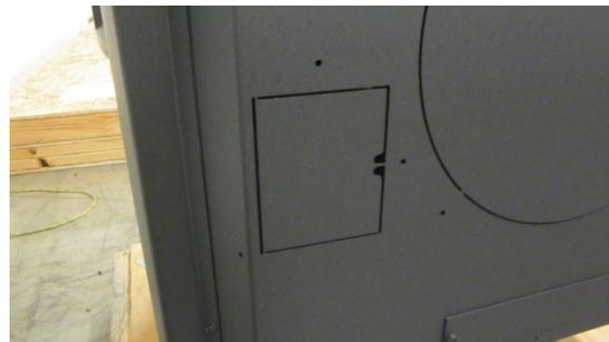
**NOTE:** On the Cape Cod (10/19 or later) the knockout is shaped like the knockout above but is located in the middle of the rear heat shield like in the picture to the left.
