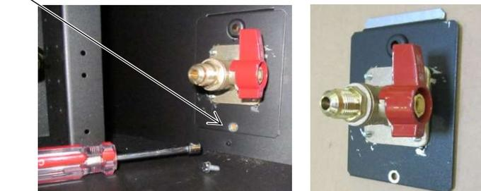
3. Remove the cover plate from the left side of the fireplace (it is held in place in the same fashion as the shutoff valve plate). Attach it to the right side of the fireplace.
