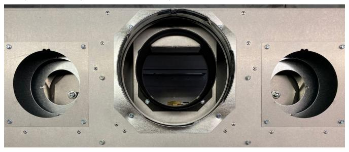
6. Insert a starter collar into each of the (2) holes that were uncovered in the previous step and bend the tabs to secure the starter collar to the fireplace. Seal the joints with silicone caulk or aluminum (U.L. 181A-P) tape.
