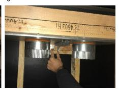
7 Insert a starter collar into each of the (2) holes that were uncovered in the previous step and bend the tabs to secure the starter collar to the fireplace. Seal the joints with silicone caulk or aluminum (U.L. 181A-P) tape.
