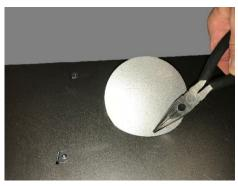
2 Grab on to the knockout with pliers and bend it back and forth until the remaining tabs break free. Discard the knock out plate.
