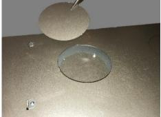
3 Under each knock out plate, you will find a cover plate held in place with (2) 1/4" screws. Use a nut driver or drill with an extension to remove the (2) screws. Reach in and remove the cover plate. You may discard the plates.
