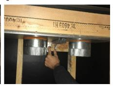
Insert a starter collar into each of the (2) holes that were uncovered in the previous step and bend the tabs to secure the starter collar to the fireplace. Seal the joints with silicone caulk or aluminum (U.L. 181A-P) tape.
