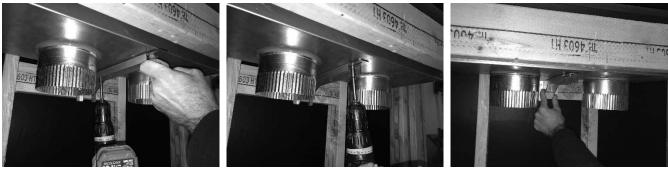
7. Stretch the included flex to its maximum length. Measure the distance between the starter collars on the fireplace and the inlets on the convection manifold. Cut the flex to the appropriate length and install between the fireplace and the manifold. Secure using (3) screws at every connection and seal the joints with silicone caulk or aluminum (U.L. 181A-P) tape.
