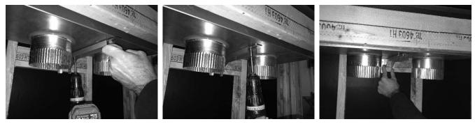
7 Remove the knockouts from the top of the fireplace (4 on the 54PB)
